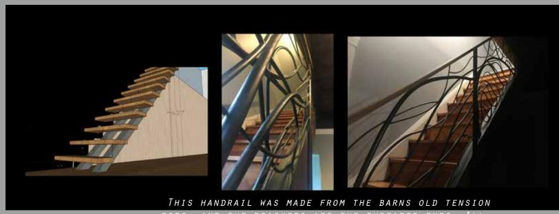
RODS, AND THE BRACKETS ARE THE THREADED ENDS. ALL PARTS WERE FORGED, RUBBED PATINA, AND WAXED. METAL AUTOMATISM TECHNIQUE
