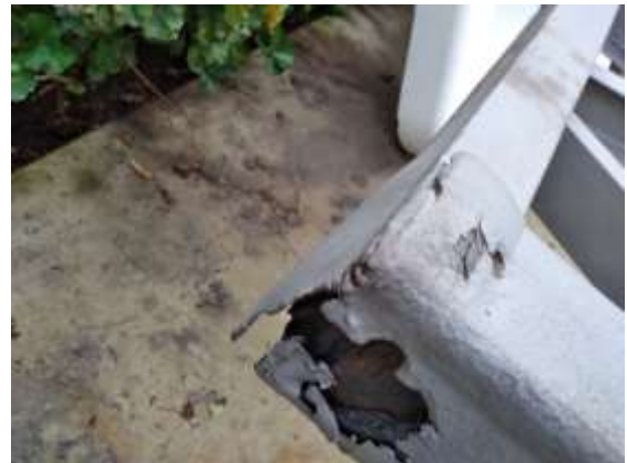
The image above is one of the many cracks and defects that Erik Chaputa will weld to get the frame ready for powder-coating. Then it's rebuilding time
