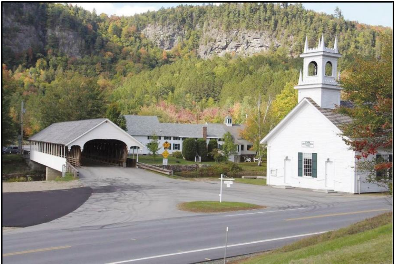
Historic Stark Union Church is facing major structural issues that require immediate attention. (BARBARA TETREAUULT PHOTO)
