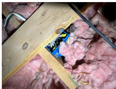
6.3 Item 2 (Picture) In attic near house fan
