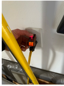
6.5 Item 2 (Picture) garage
