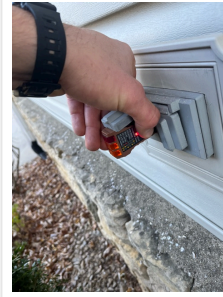
6.5 Item 3 (Picture) garage exterior
