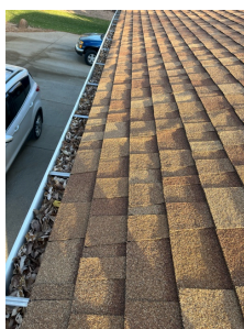
1.3 Item 1 (Picture) north side gutter
