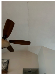
3.4 Item 2 (Picture) Ceiling in entry way/kitchen
