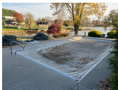
12.0 Item 1 (Picture) pool
