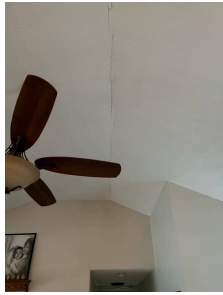
8.0 Item 1 (Picture) entry way ceiling
