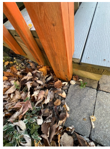
2.3 Item 5 (Picture) west deck post
