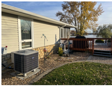
4.8 Item 1 (Picture) Outdoor condenser unit
