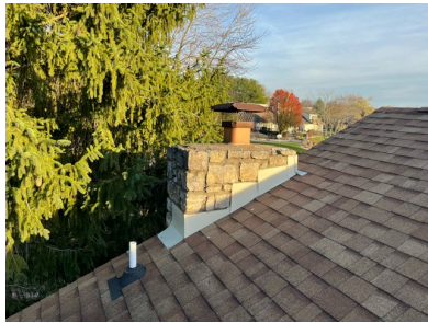
1.2 Item 1 (Picture) Chimney
