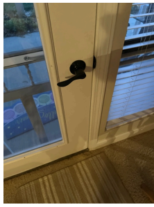
2.1 Item 1 (Picture) Basement exterior door
