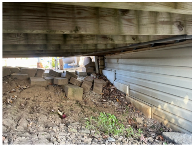
2.3 Item 4 (Picture) underside west deck
