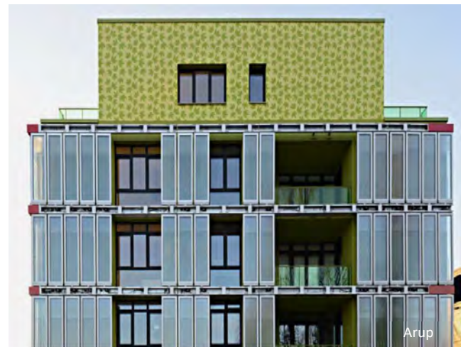
Bio Intelligent Quotient House in Hamburg, Germany with its 'SolarLeaf' façade of flat panel glass bioreactors containing microalgae that produce bioenergy and heat for the building.
