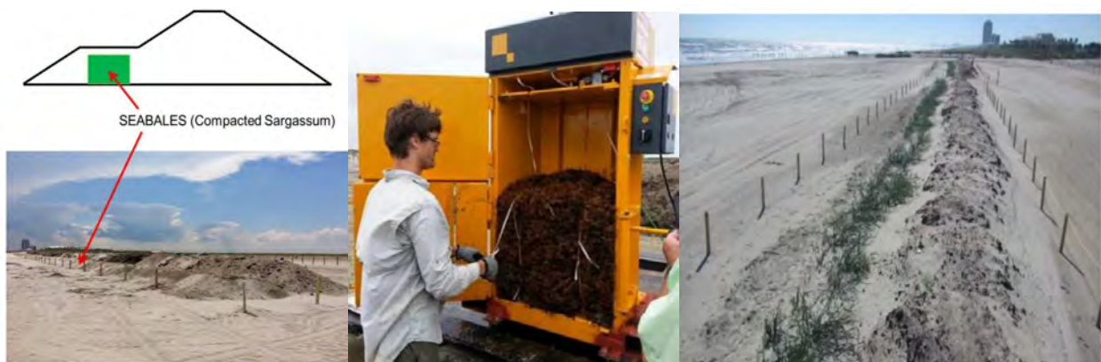
Pelagic sargassum 'Seabale' project for dune restoration on Galveston Island, conducted by Texas A&M University. Source: Figlus et al. (2015).
