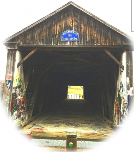
The bridge as it stood.
