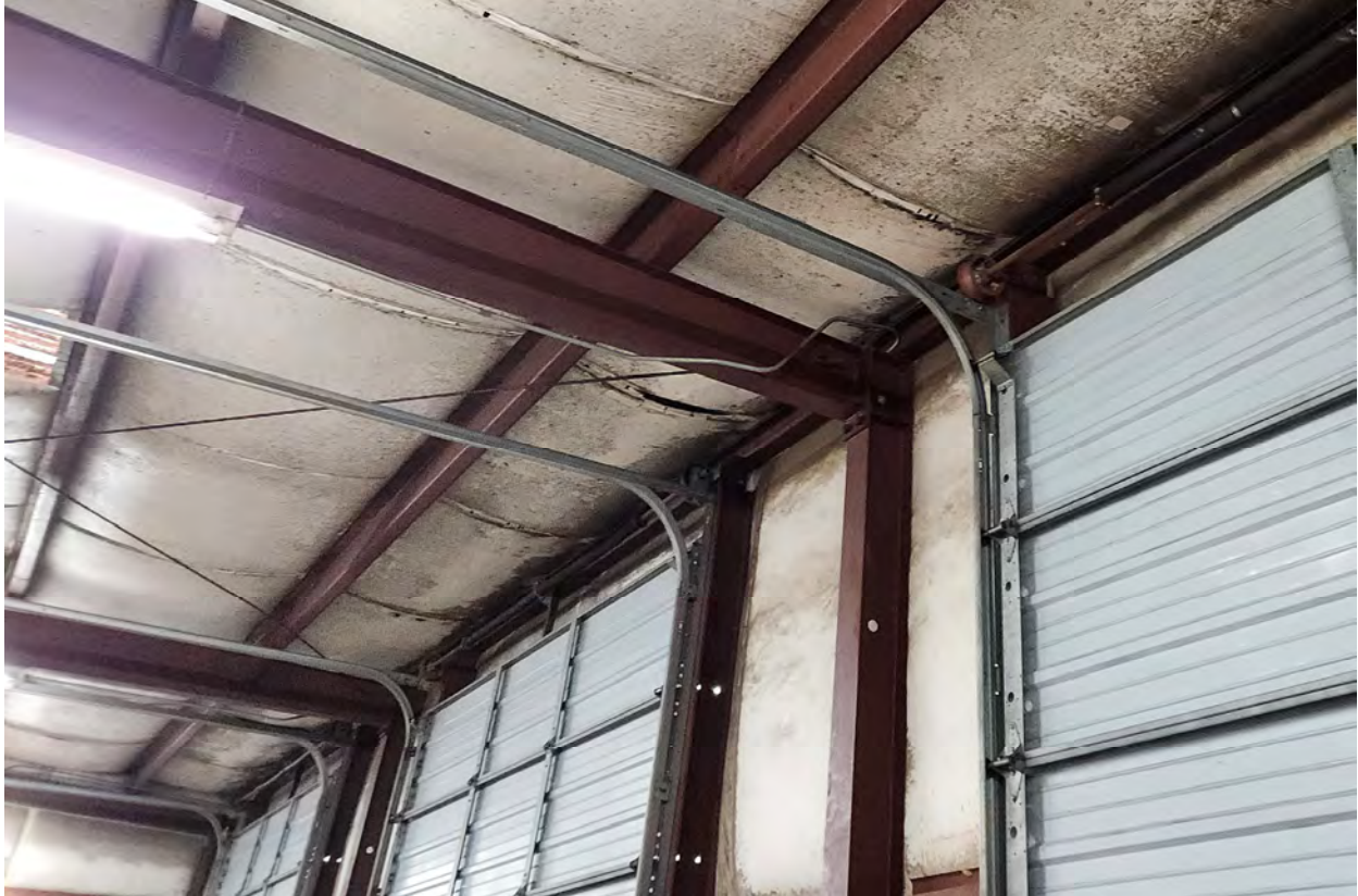
4.3 Building Envelope: The buildings are clad with metal panels.
