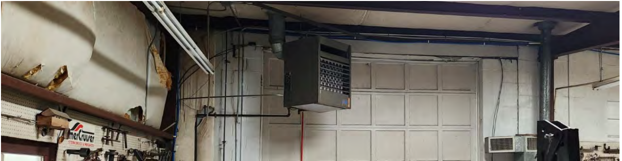
North Rear Building: Heated with an overhead gas heater.
