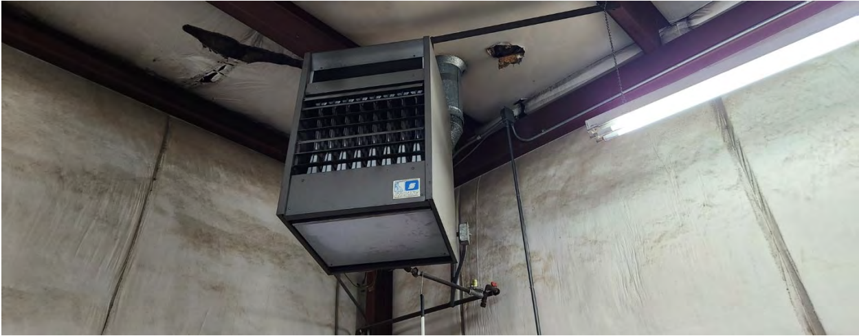
North Rear Building: Heated with an overhead gas heater.
