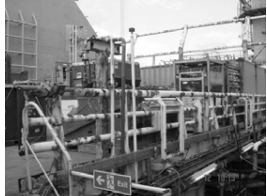
FIGURE 2: Small intricate areas for repair
