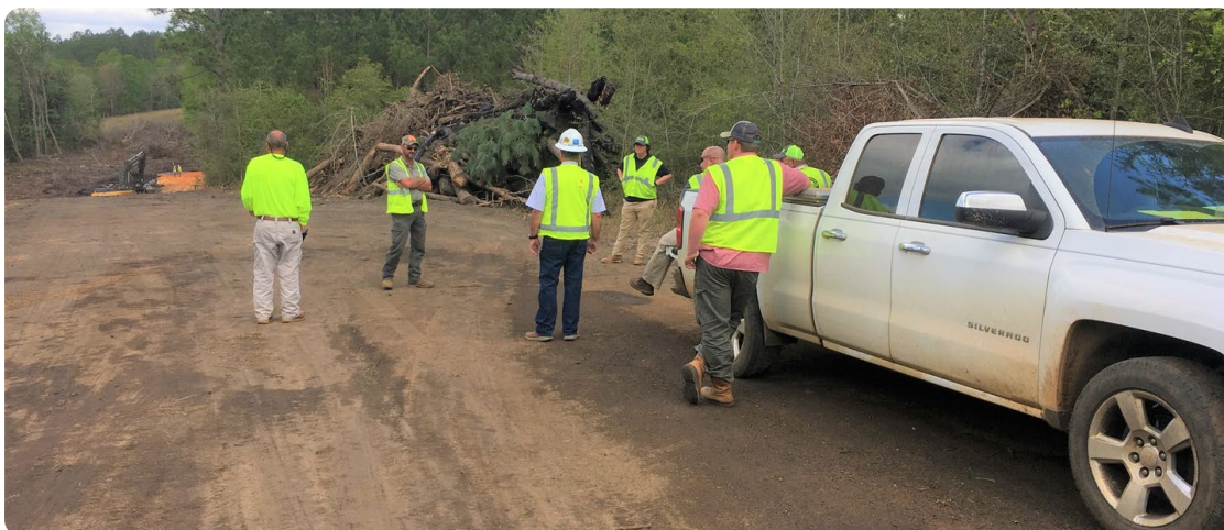
Joey Fresolone leads a weekly socially distanced project meeting with a contractor and project staff.
