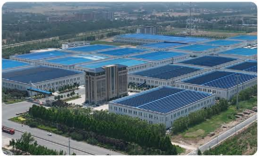
BIOBASE Juancheng County Medical Equipment Industrial Park
