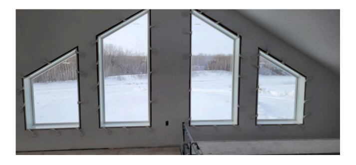
Rake Head windows are more complex and leave more room for error when attempting to order a jamb that will slide right into place. Due to the complexity, we only sell lengths of material that can be cut to length and assembled on site.
