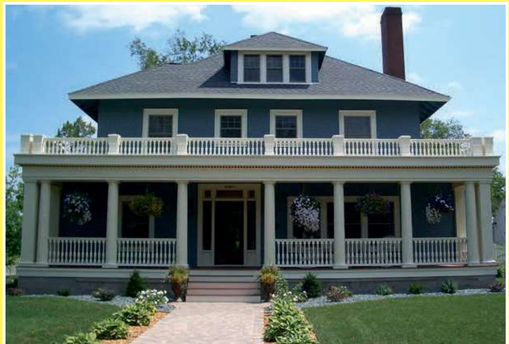
Photo above shows the use of Spectis balusters, top & bottom rails, custom newel posts & caps and columns with caps & bases
