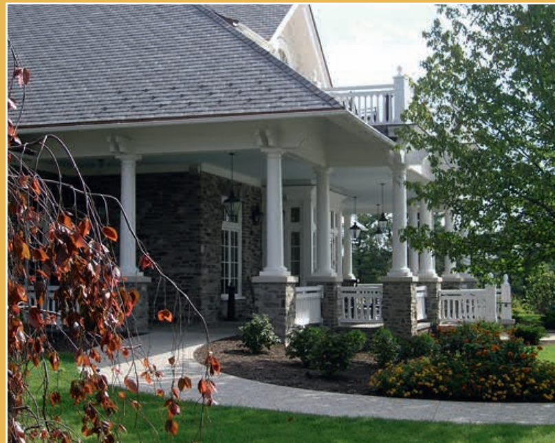
Photo above shows Spectis columns with cap & base, balusters, top & bottom rails, and newel posts with cap and ball top
