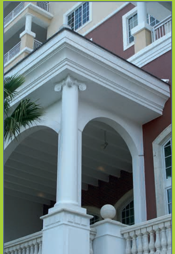
Photo above shows use of Spectis custom moulding and columns with cap & base
