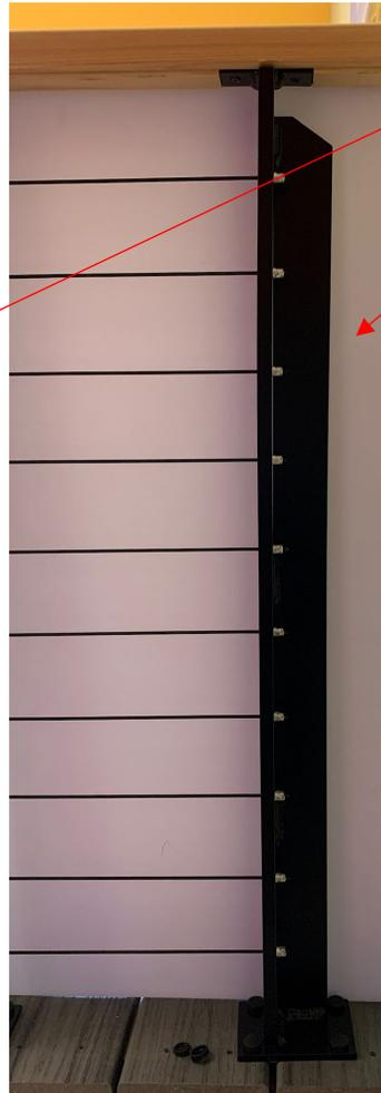
The post in the left photo should be reversed 180 degrees to have the solid bar cover the crimped ends. This would make for a much cleaner look. The post in the right post is correct, the crimps are behind the solid bar.
