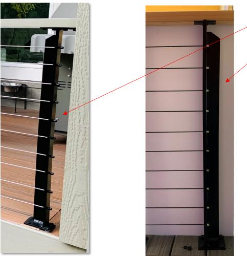
The post in the left photo should be reversed 180 degrees to have the solid bar cover the crimped ends. This would make for a much cleaner look. The post in the right post is correct, the crimps are behind the solid bar.
