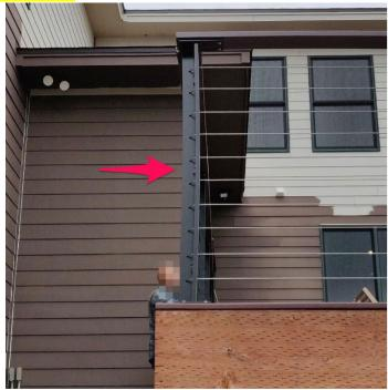
In this case, you might be replacing cables and possibly even a top cap. When tensioning cables, a little goes a long way. If your cables are too tight, then you will have to cut them and get a new set. There is no way to back off the tension on the one-way valves. So be careful to not go too far.
