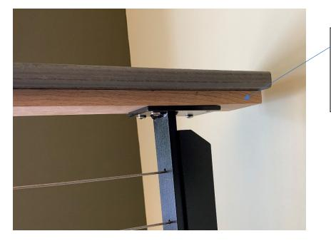
Our wide top posts require a 1x4 of oak or similar material. You need a strong wood to keep the screws from tearing out of the wood. Your decking goes on top of the 1x4 oak.
