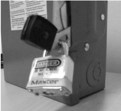
Figure 3 Typical Locking Disconnect Switch
