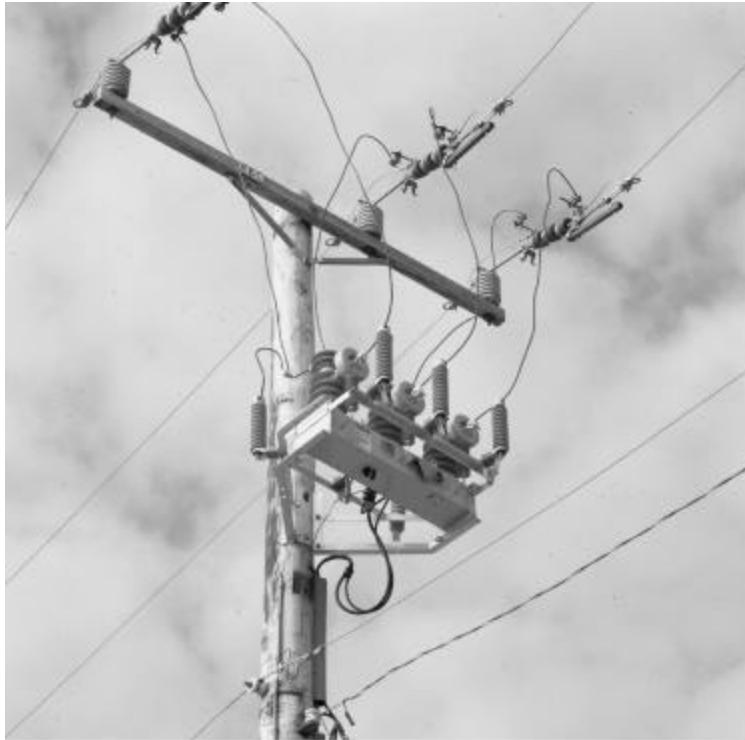
Figure 5-52: Mounted Recloser. Courtesy of Cooper Power Systems.
