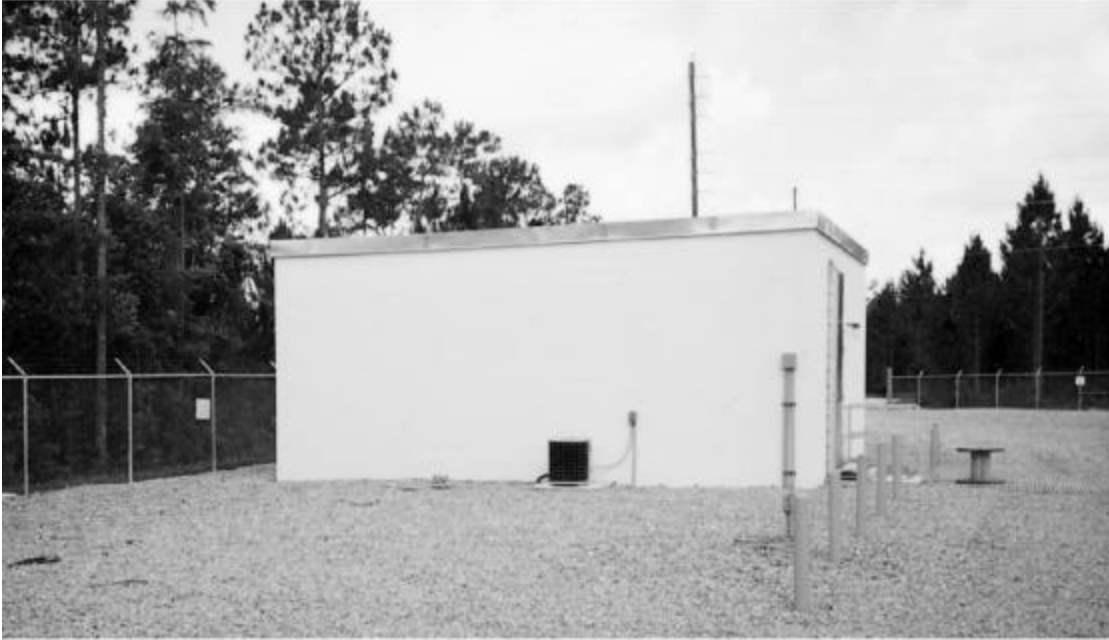
Figure 16-2: Typical Masonry Block Control Building
