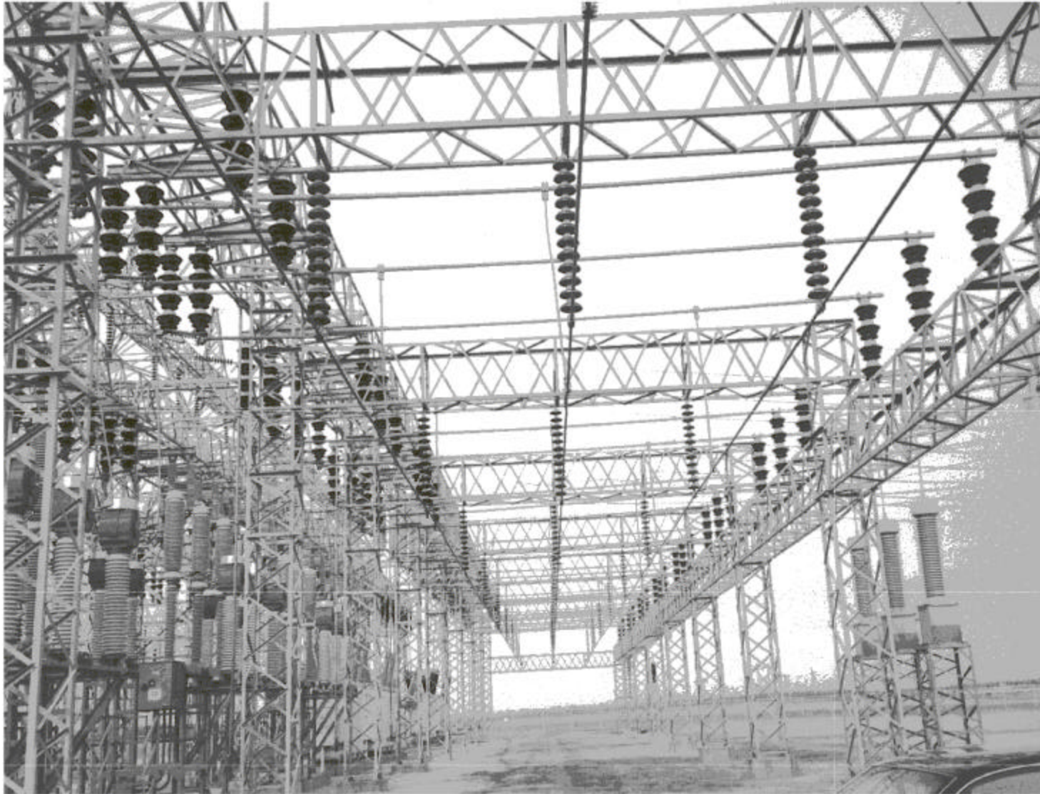
Figure 4-20: Suspension Insulator
