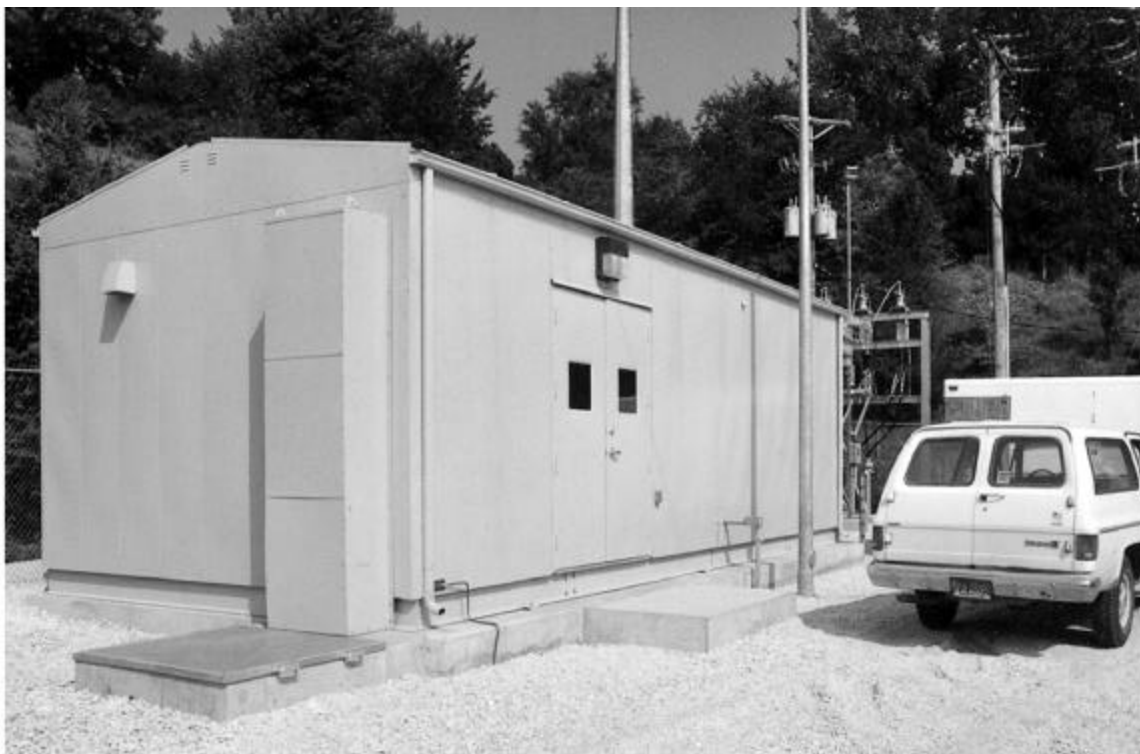
Figure 16-1: Pre-Engineered Metal Control Building (Coffeyville, KS)
