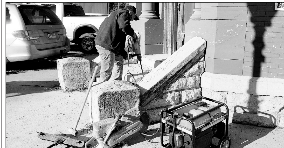
New stone steps were recently installed at the entrance of the Old Bank Museum which is a Jefferson County Historical Society site. Grant dollars from the Diller Community Foundation Fund helped cover project costs. Painting to the exterior of the building was completed and offered a welcoming appearance to guests who toured the displays during the 124th Diller Picnic weekend, June 17 - 19.
