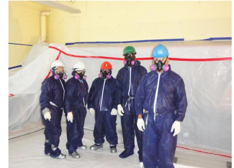
PCBs were added to caulk and elastic sealant materials, particularly from 1950-1977. When caulk with PCBs is disturbed, it may produce dust that contains PCBs. The SCA has developed and implemented stringent dust control practices to minimize the potential exposure to PCB-containing dust during construction.
