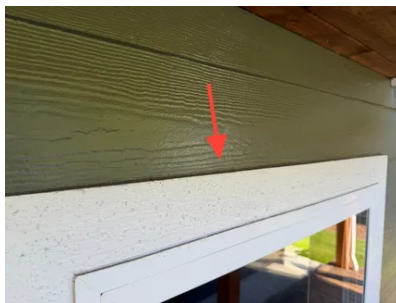
This shows a proper head flashing.
