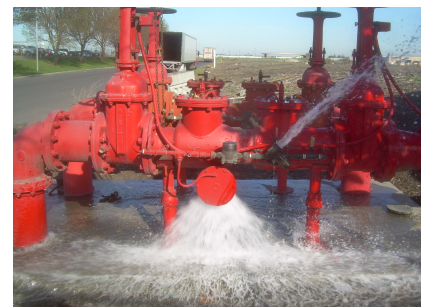
Full relief valve discharge
