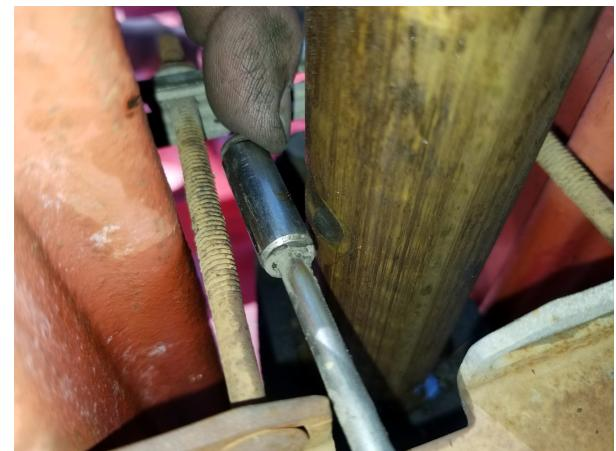
**Step #2:** After I'm done testing and I have opened the gate valve and the motion detector arm is back in the groove, I repeat the procedure to insure that I can hear the same number of clicks that I did in Step #1.
