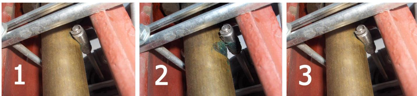
**1:** The arm rests in a groove on the gate valve stem when the gate valve is open.
