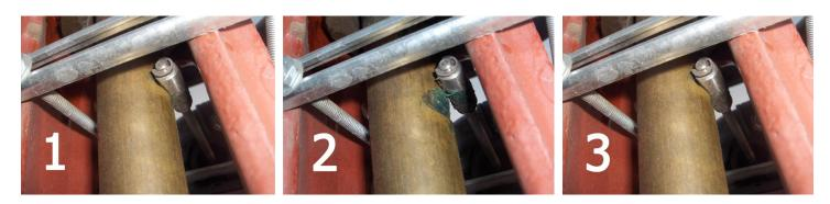
**1**: The arm rests in a groove on the gate valve stem when the gate valve is open.
