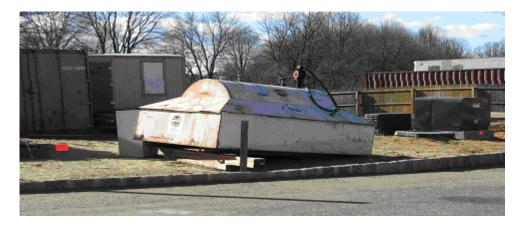
This fuel storage should have a secondary pan as a backup in the event of leakage.
