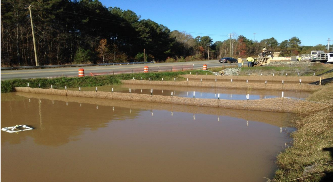
9.8 skimmer baffle area before FLOC treatment
