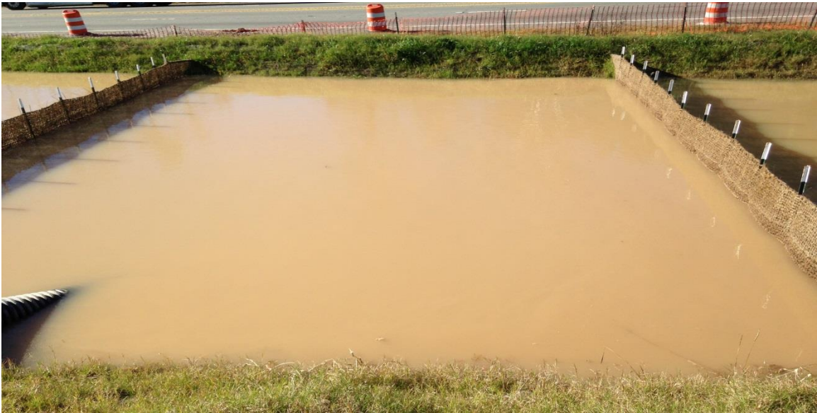
9.8 basin 45 minutes after FLOC application
