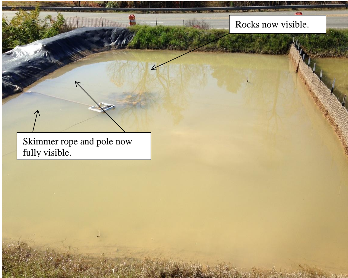
9.8 skimmer baffle area at 11:17 a.m. the following day 11/21/15
