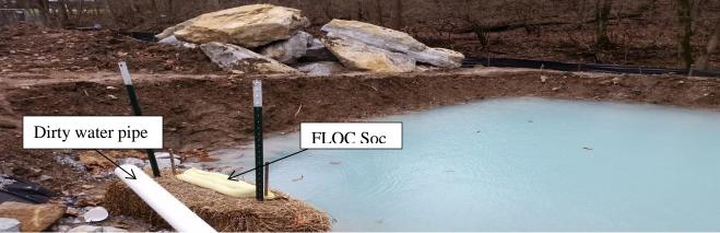
**Maintenance:**FLOC Soc now being used to dose the FLOC into the basin instead of hand dosing. The dirty water being pumped into the basin comes out the white pipe directly onto the FLOC Soc releasing the FLOC slowly out of the FLOC Soc.
