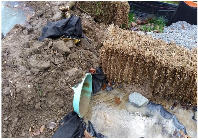
Water now draining from last baffle area clear at 11:14 a.m. .5 hours after FLOC application. (Discharge pipe into creek)
