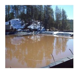
Lewis Pit Reservoir Being Treated with FLOC Socs
