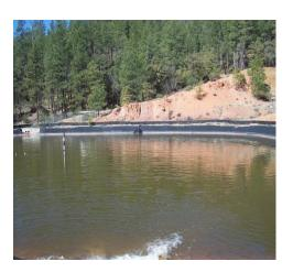
From the Lewis Pit Reservoir, the FLOC treated water at 4.6 NTU was then treated with the remainder of the FLOC Socs and filtered through the R-4 Treatment Plant which consists of 2 parallel sand filter tanks, one ½ micron 22 cartridge canister and two banks of UV lights. Water was circulated for 48 hours over the FLOC Socs and through the R-4 Treatment Plant. Final turbidity was 1.5 NTU.
