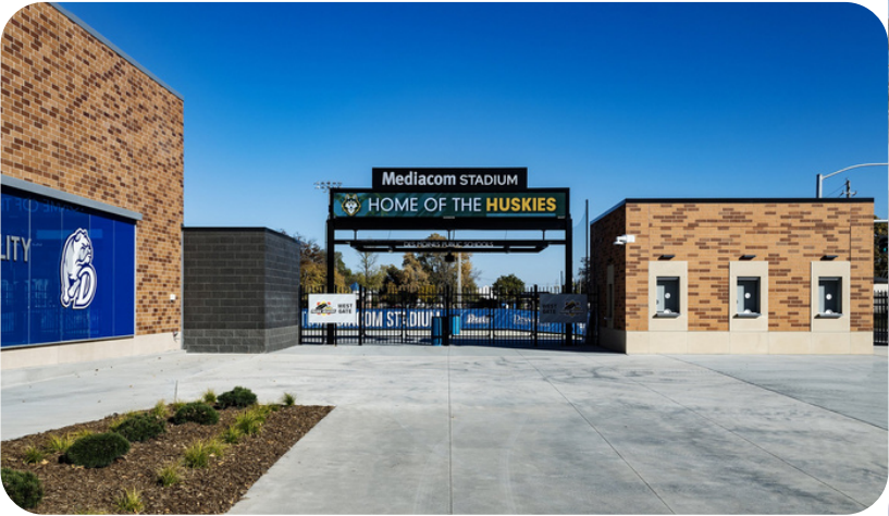
WEST GATE ENTRANCE
