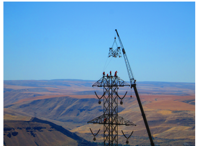
Major upgrades to the country's transmission lines are included in infrastructure legislation.
