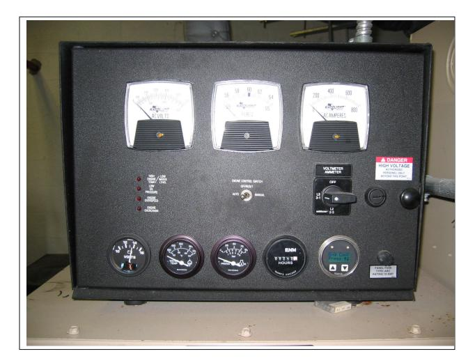
To shut down or keep the Generator from starting put the ENGINE CONTROL SWITCH in the middle position, <u>OFF/RESET</u>. If the generator was running it will take several minutes for it to stop.
