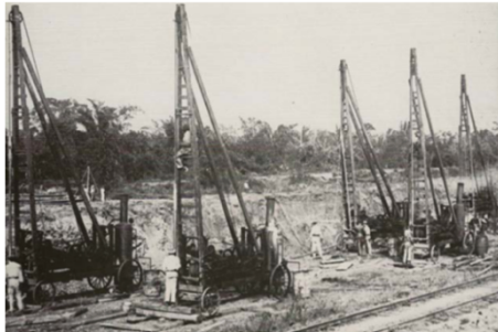
Tripod pneumatic drills in the Panama Canal, 1907.
