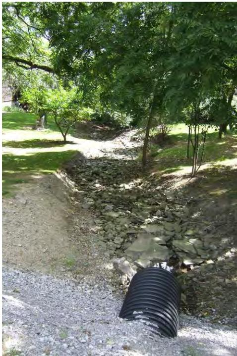
View of culvert and riprap stabilization looking downstream from Bacon Rd. Bare soils can be seen on the left bank and mowed grass is adjacent to top of banks on both sides.
