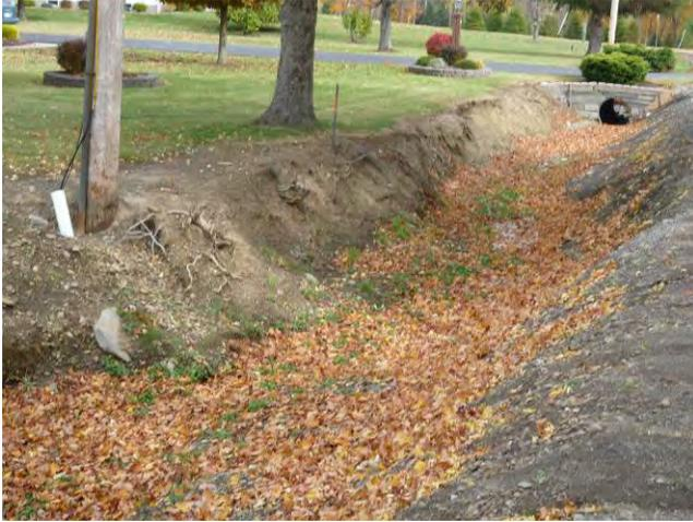
A view of the channel between the second and third properties. The telephone pole is becoming exposed, tree roots are visible. Both banks are experiencing severe erosion.
