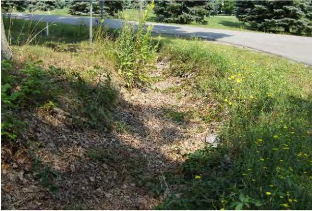
The corner of Silver Grove and Luther Rd. Erosion of the inner bank can be seen as well as rock rip rap used to stabilize the bank.
