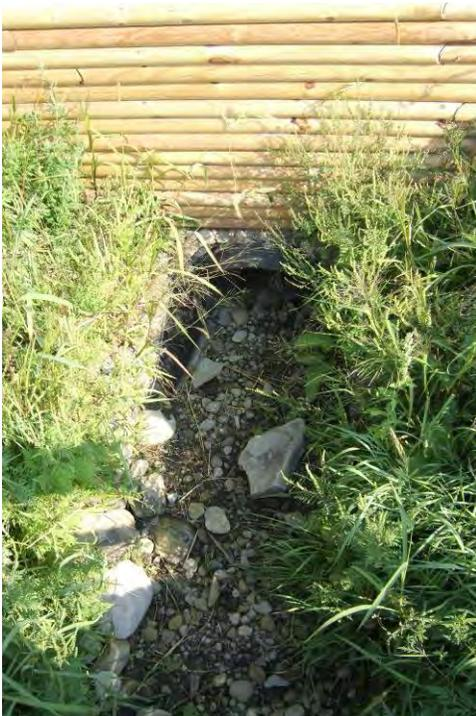
Gravel and sediment in end section of culvert indicating moderate erosion in upstream channel.
