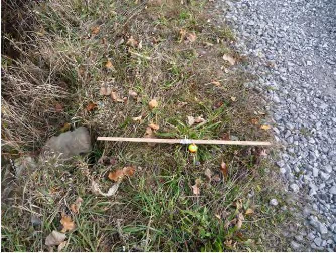
Portion of the channel where the bank is less than 3 ft from the roadway.
