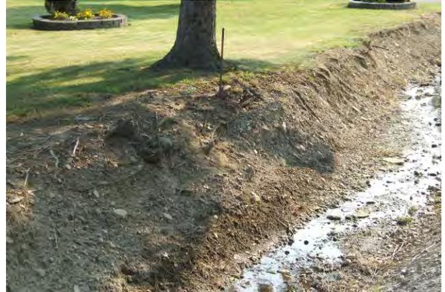
Part of the channel between the second and third properties. Water has cut into the far bank approximately 6 inches to 1 ft deep. The telephone pole is to the immediate right of the photo.
