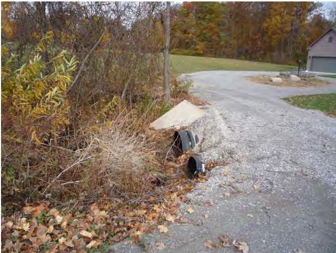
Driveway crossing suffering from erosion. Rill can be seen on the sides of the drainage pipes and a concrete slab was placed along the far bank to help stabilize the bank.
