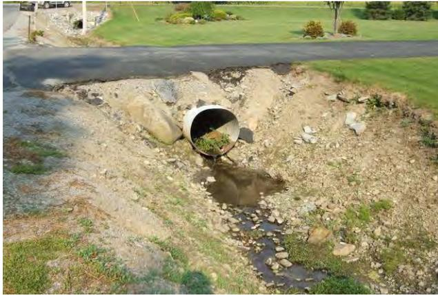
View of the first driveway crossing outlet. Similarly, stabilization has been attempted. Erosion can be seen on both banks from the road and the driveway.
