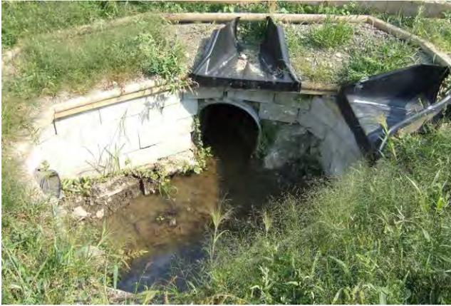
Culverts and end sections with minor erosion around buried culvert pipe
