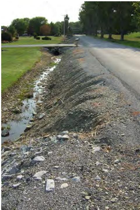
Looking downstream from the culvert outlet. Rock rip rap and deep rills can be seen in the roadside bank.
