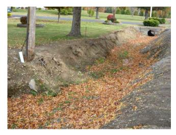
A view of the channel between the second and third properties. The telephone pole is becoming exposed, tree roots are visible. Both banks are experiencing severe erosion.
