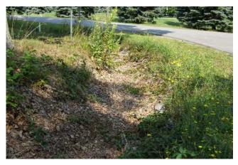
The corner of Silver Grove and Luther Rd. Erosion of the inner bank can be seen as well as rock rip rap used to stabilize the bank.
