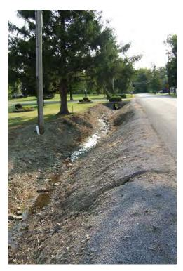
A view of the channel between the first and second properties. The second driveway crossing can be seen. Steep bank grade and rilling can be seen. The far bank, lacking vegetation, is also seen.
