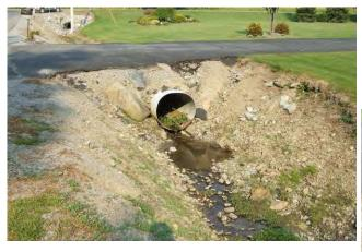
View of the first driveway crossing outlet. Similarly, stabilization has been attempted. Erosion can be seen on both banks from the road and the driveway.
