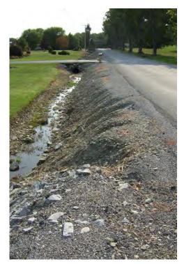
Looking downstream from the culvert outlet. Rock rip rap and deep rills can be seen in the roadside bank.
