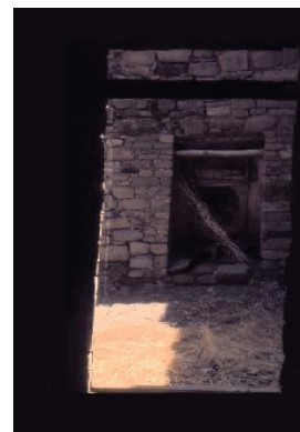
Right, multiple sets of aligned interior doors like the three here are another iconic feature of this complex site.
