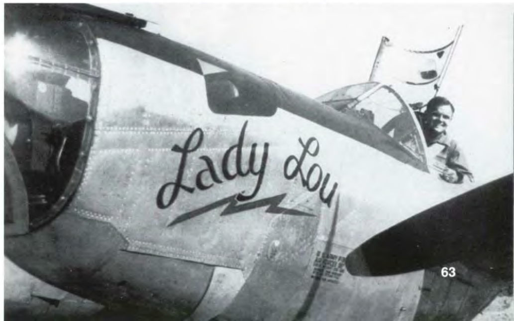
Lady Lou was a P-38J 'Droop Snoot' assigned to the 82nd FG at Vincenzo Airfield, Italy in early 1945. This aircraft lacks the narrow Plexiglas window just aft of the nose bubble, but retains the larger window further back. 'Droop Snoots' led fighter aircraft formations on high altitude horizontal bombing attacks. All aircraft in the formation dropped their bombs on the 'Droop Snoot' bombardier's command " Bombs away! " (USAFM)
