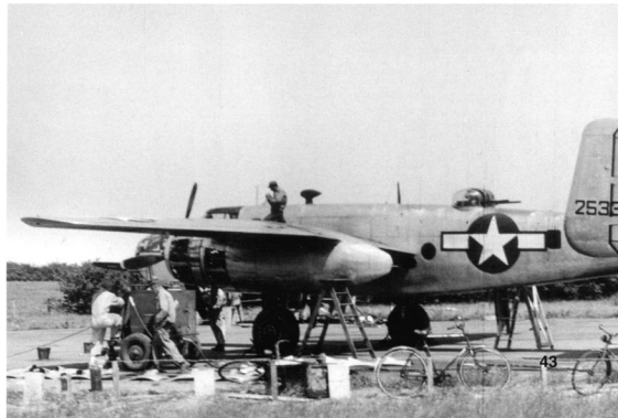
B-25C-5-NA (42-53357) of the 7th Photo Group undergoes field maintenance at Mt. Farm Airfield, England during 1945. For defensive purposes it retains the dorsal turret (though the retractable ventral turret is missing) and a nose gun. (Robert Astrella via Norm Taylor Collection.)
