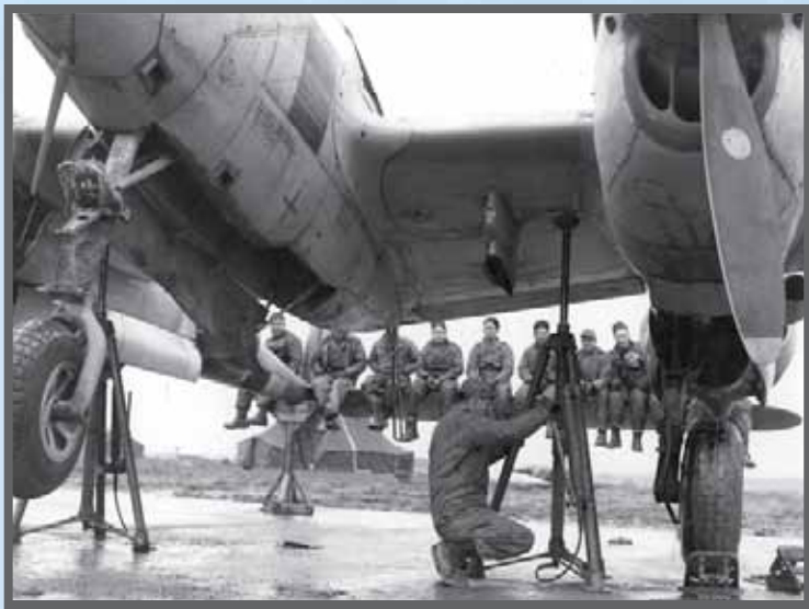
Airmen sit on tail of P-38 Lightning to lift its nose wheel for landing gear maintenance.
