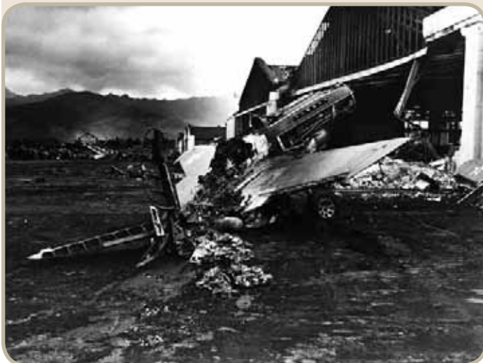
Damage at Wheeler Field.
