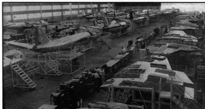
For the production of the B-57, Martin moved back into their former government-owned World War II B-26 Marauder assembly plant No 2 across the road from their main facility. RB-57As are shown in various stages of production. Navy personnel served as purchaser and handled administrative matters for the US Government and USAF at the Martin plant. (Martin)
