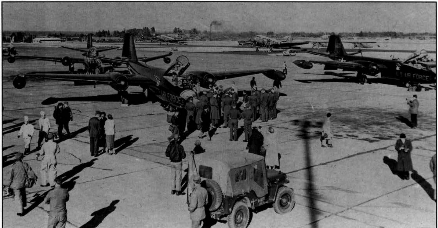
On 9 January 1956, the first B-57s arrived at Johnson AB, Japan, for the 3rd Bomb Group. Their former B-26 crews were sent from Japan to Randolph AFB for training, then to ferry their new bombers to their home station in Japan. Frequent groundings of the Canberra in these early days heavily disrupted this scheduling.
