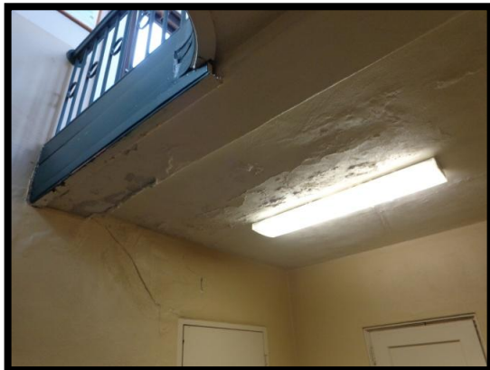
Cracking in Basement Walls & Ceilings
