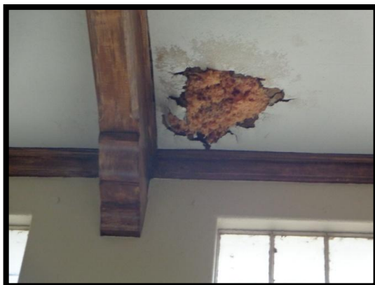
Water Damages in Main Hall Ceiling
