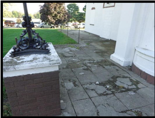
Deteriorating Westside Terrace
