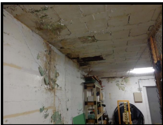
Water Damage in Basement Storage Room
