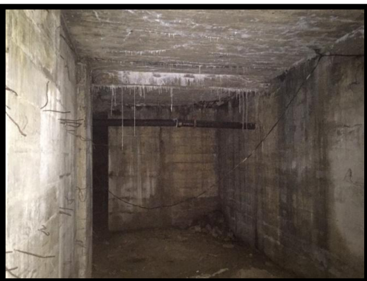
Water Damage Under Westside Terrace
