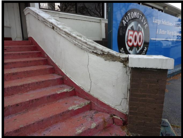
Deteriorating Steps on the East Side
