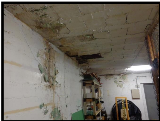
Water Damage in Basement Storage Room
