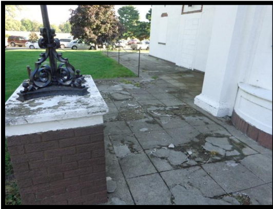
Deteriorating Westside Terrace
