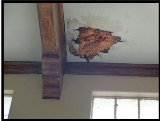
Water Damages in Main Hall Ceiling
