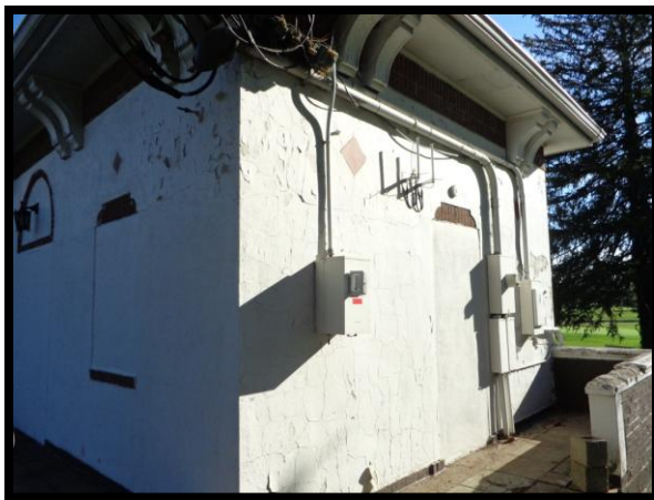
Outside Electrical Boxes
