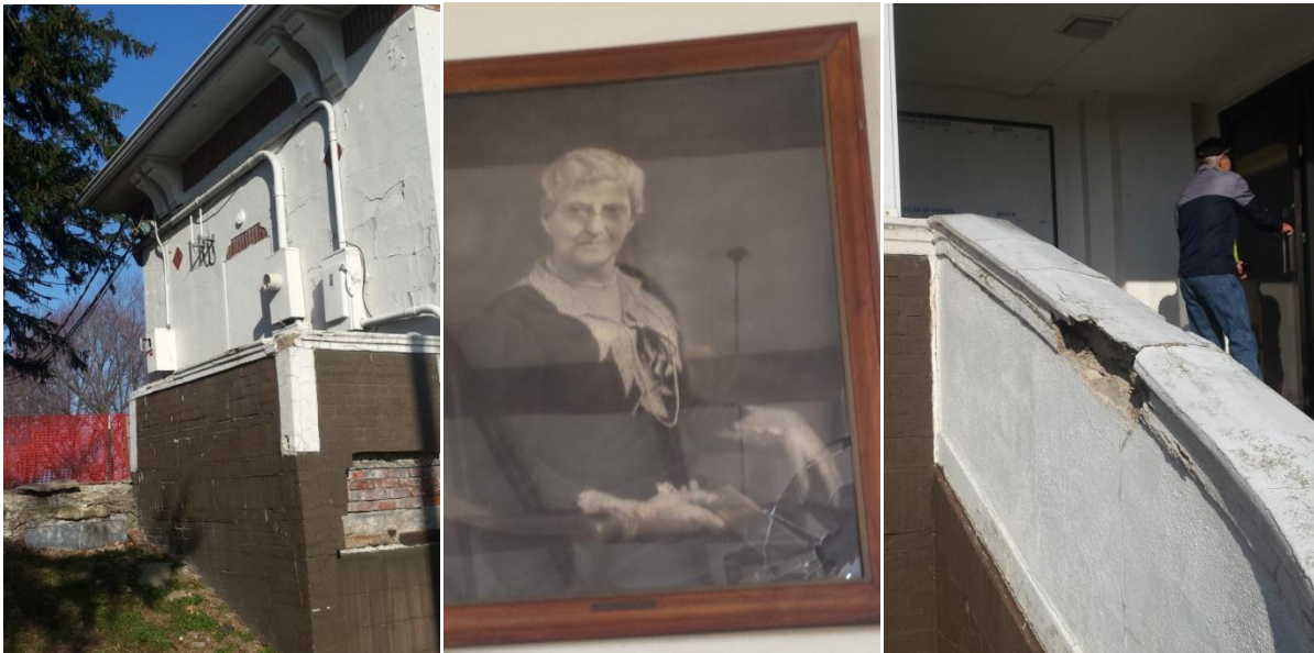
L to R: South side of clubhouse, Mrs. Rea's damaged portrait, crumbling east side stairway
