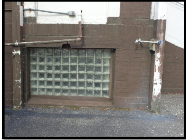
Outside Water Lines
