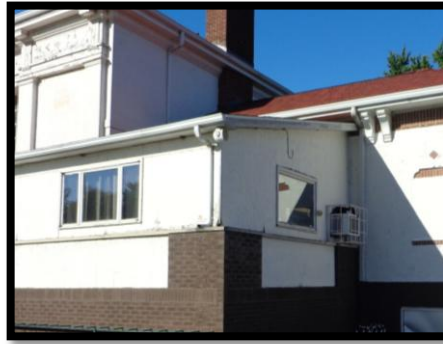
Pro Shop Window A/C
