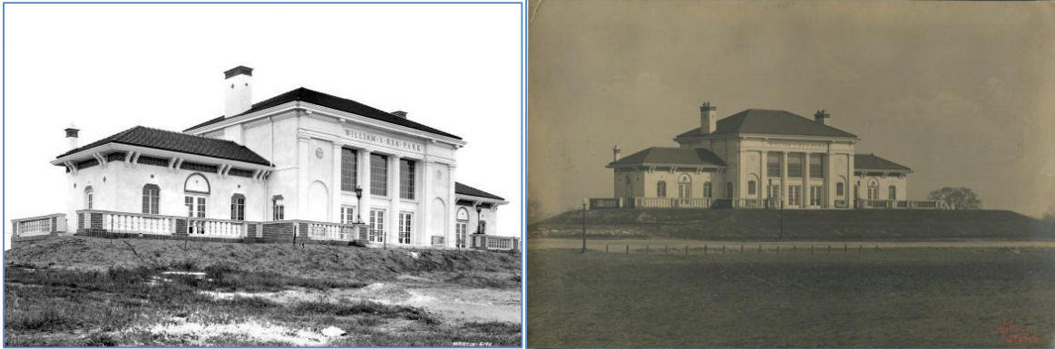
L to R: Clubhouse under construction and shortly after completion in September 1925
