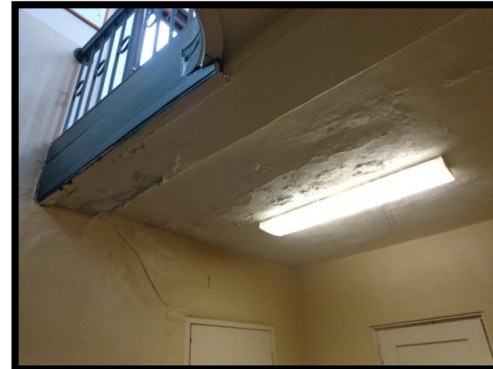
Cracking in Basement Walls & Ceilings
