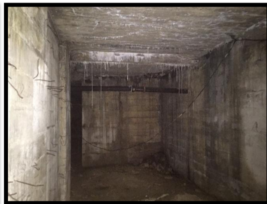
Water Damage Under Westside Terrace
