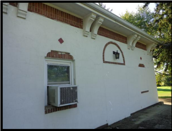
Windows Blocked Shut
