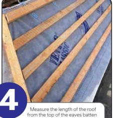
Measure the length of the roof from the top of the eaves batten to the apex of the roof from the total then divide this figure by 200mm (the maximum gauge of the Cromaslate) e.g. if the length of the roof is 3695mm, minus 25mm = 3670mm divide by 200mm = 18.35. Always round this number UP to the nearest full number 19 and then divide the 3670mm by 19 = 193mm this will be the gauge of the batten from the top of one to the top of the next.
