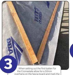
underlay at 250mm either end of the roof.
