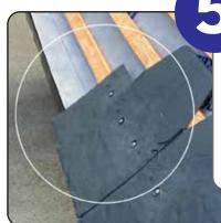
Once all the underlay and battens have been fixed into place cut the eaves slates to a length of 300mm by using a hand saw or similar. If it is a straight up and over roof start at the verge allowing the correct overhang on the verge and the 50mm over the fascia/ eaves ventilation. Fix the eaves slates into the batten using the appropriate nails/screws.
