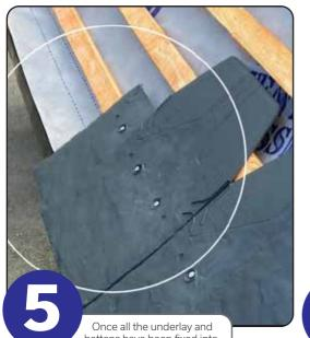
battens have been fixed into place cut the eaves slates to a length of 300mm by using a hand saw or similar. If it is a straight up and over roof start at the verge allowing the correct overhang on the verge and the 50mm over the fascia/ eaves ventilation. Fix the eaves slates into the batten using the appropriate nails/screws.
