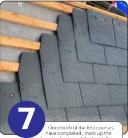
have completed, mark up the from the bottom of the first full slate to what the gauge of the slates are ,using a blue chalk line strike a line across and this will give you a mark to keep the slates straight.
