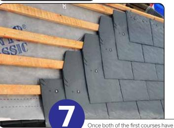
completed, mark up the from the bottom of the first full slate to what the gauge of the slates are ,using a blue chalk line strike a line across and this will give you a mark to keep the slates straight.
