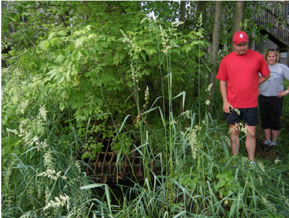
Photograph No. 1 - View south at storm water outfall located between Lots 16 and 17
