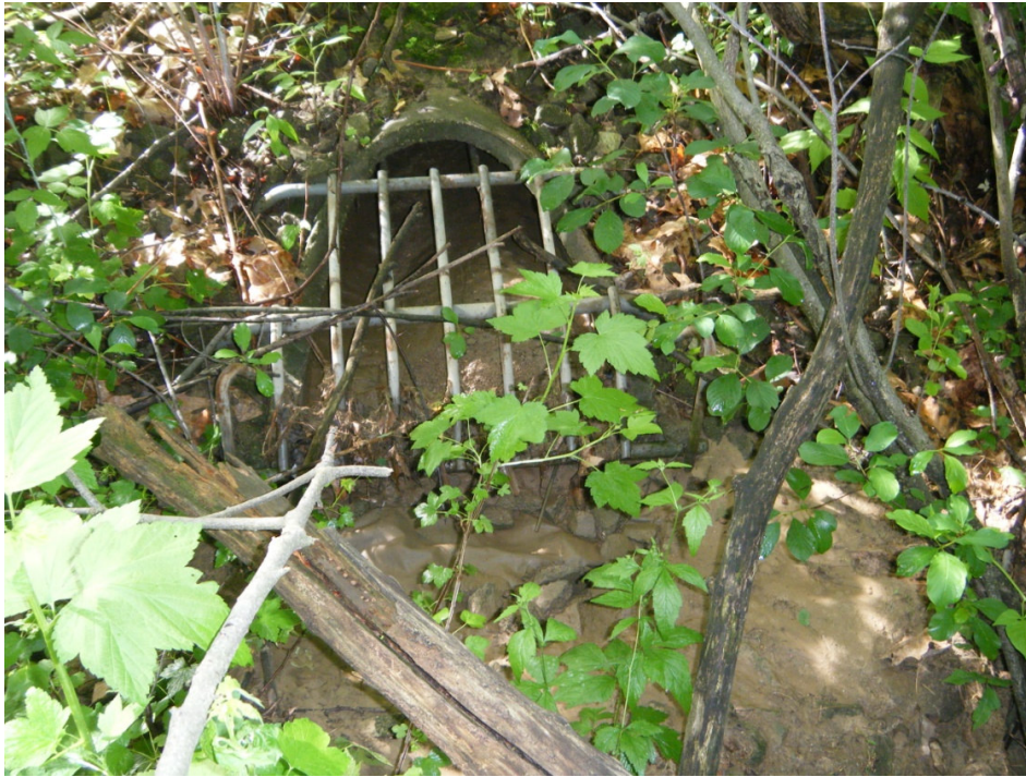
Photograph No. 9 - View south at storm water outfall located between Lots 51 and 52
