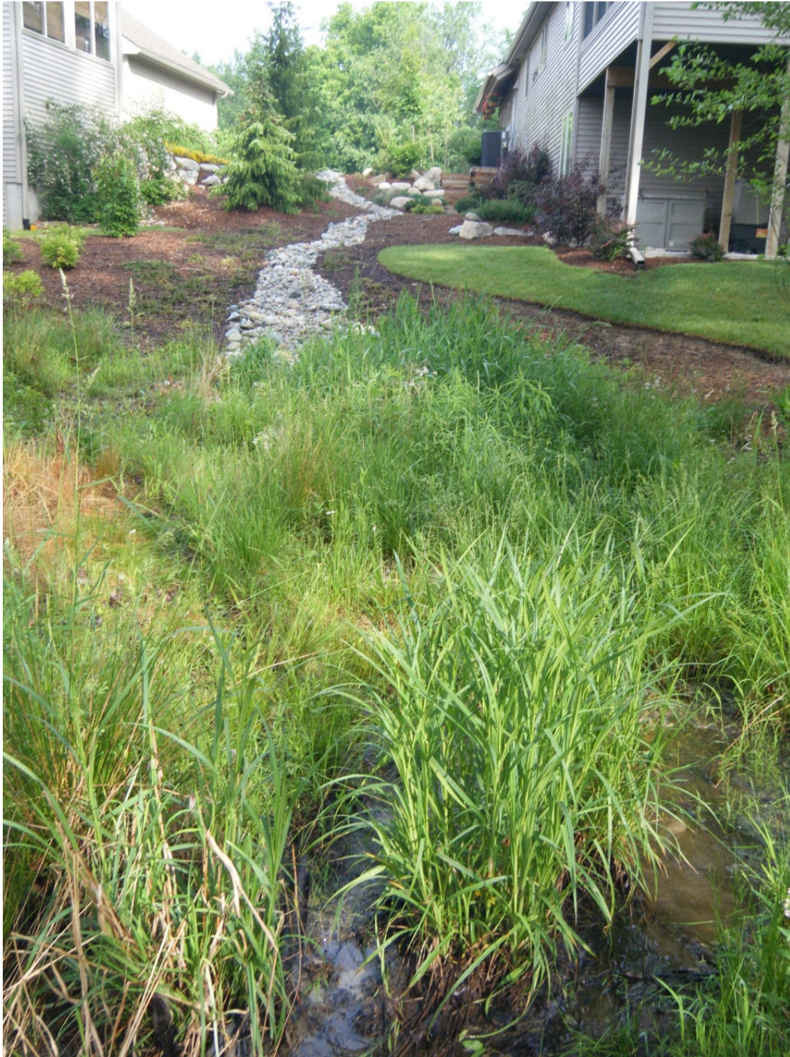
Photograph No. 5 - View northwest at storm water outfall located between Lots 126 and 127
