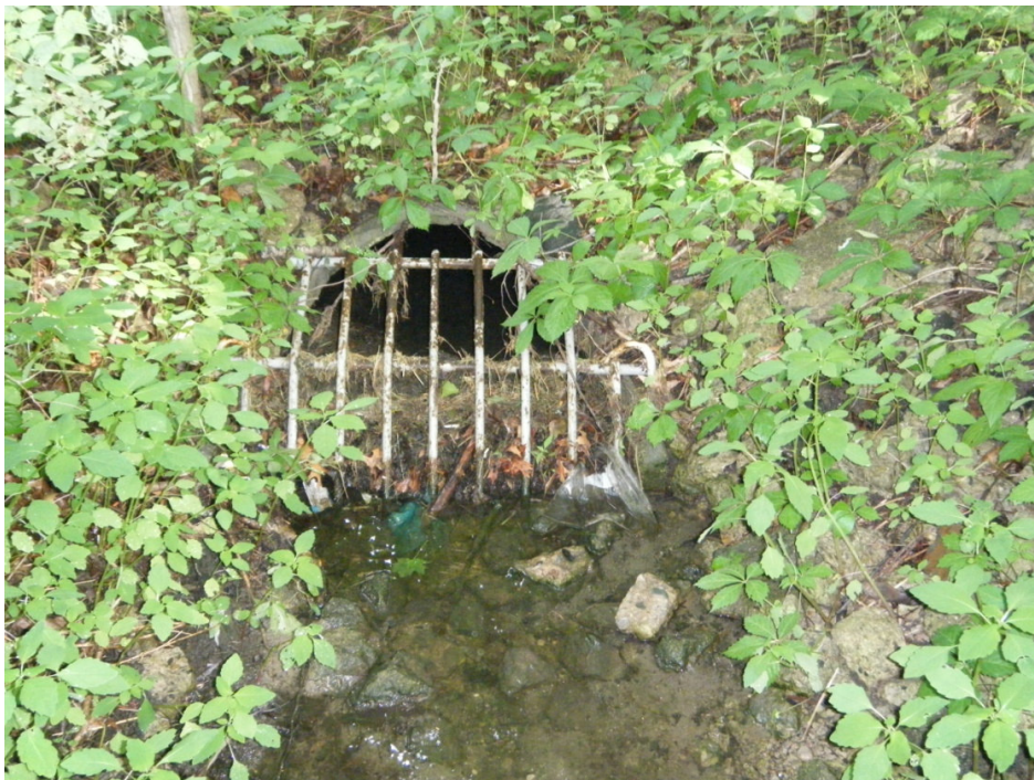
Photograph No. 10 - View northwest at south end of equalization culvert located north of Lots 29 and 30
