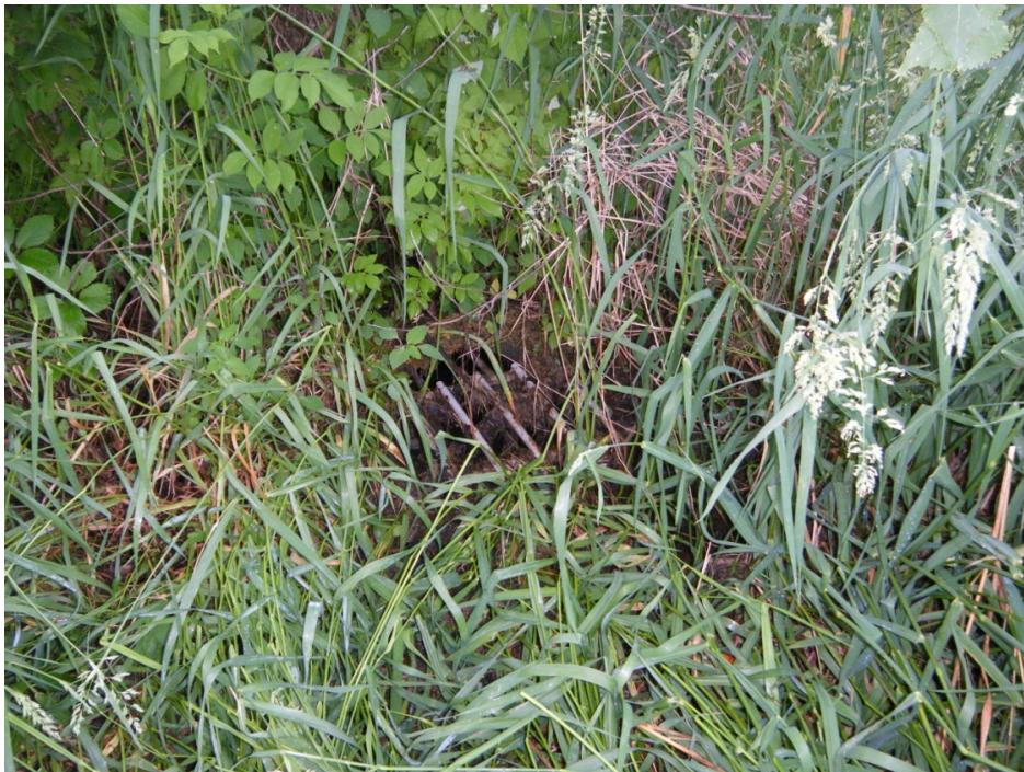
Photograph No. 2 - View east at stormwater outfall located south of Lot 8 (Note: blockage within outfall and heavy growth of vegetation at discharge point)
