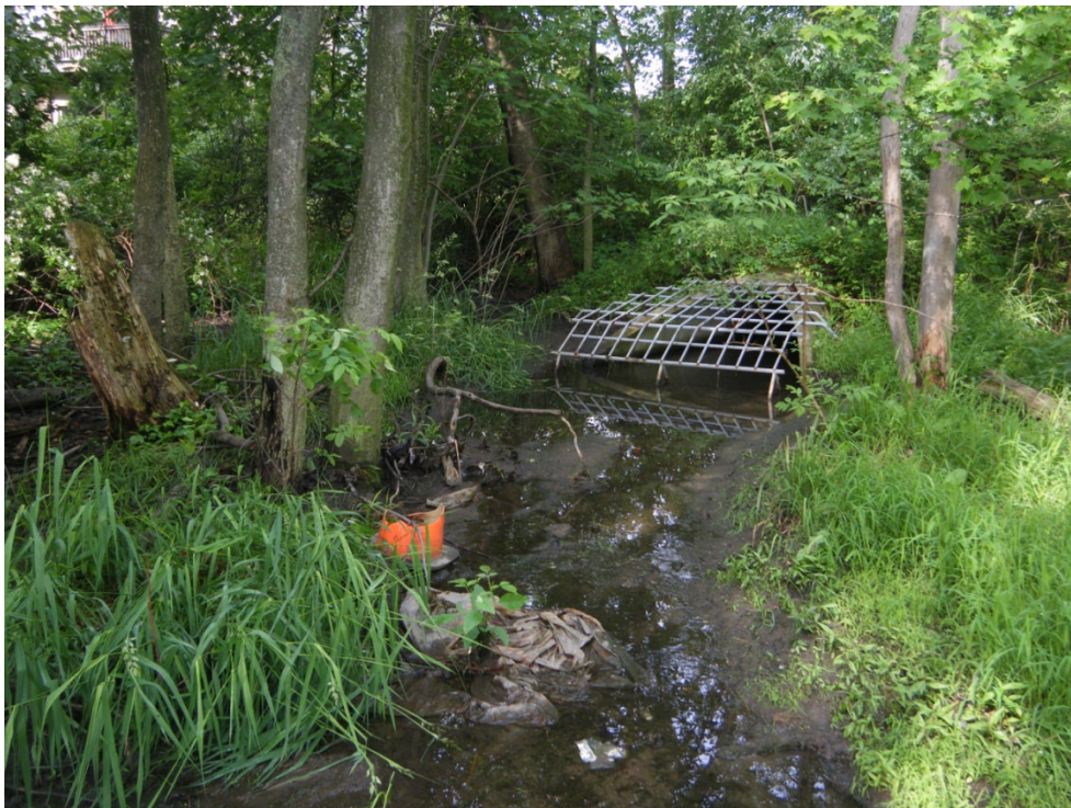
Photograph No. 7 - View southwest at storm water outfall located between
