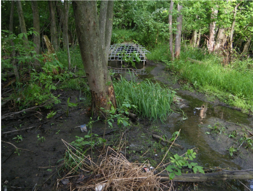
Photograph No. 6 - View west at storm water outfall located between Lots 137 and 138
