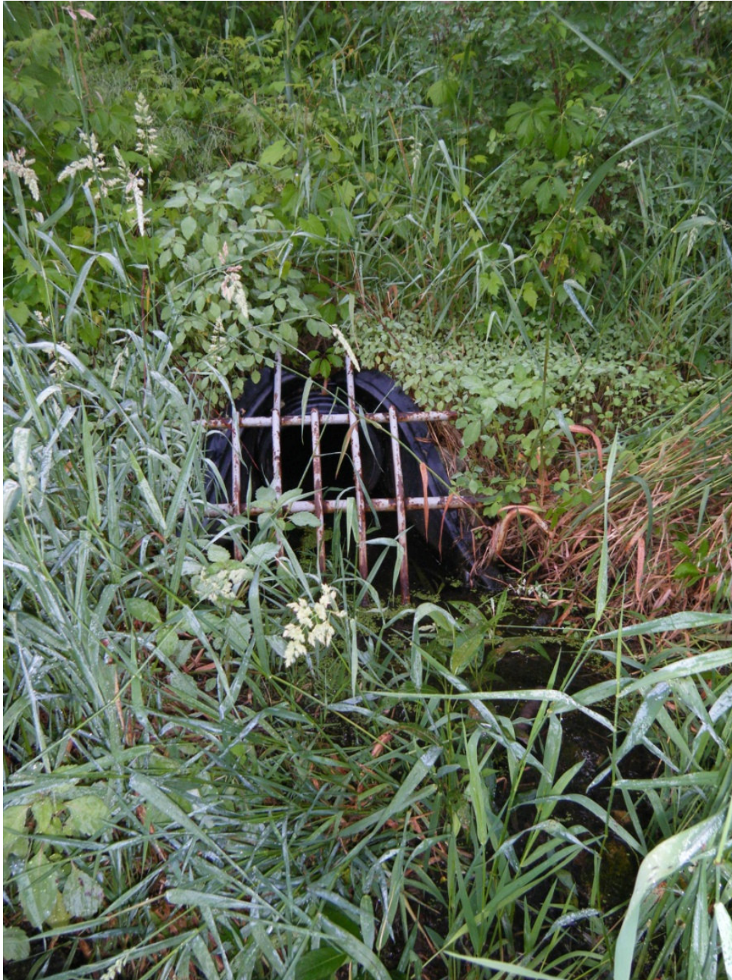
Photograph No. 3 - View east at outfall located north of Lot 14
