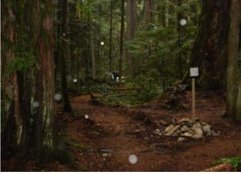
October 21, 2011 - The machine gets to the end to the pad for wheelchair turn around. On way out it will smooth trail. Next is compressing and crusher dust hauled in and compressed - lots of work.
