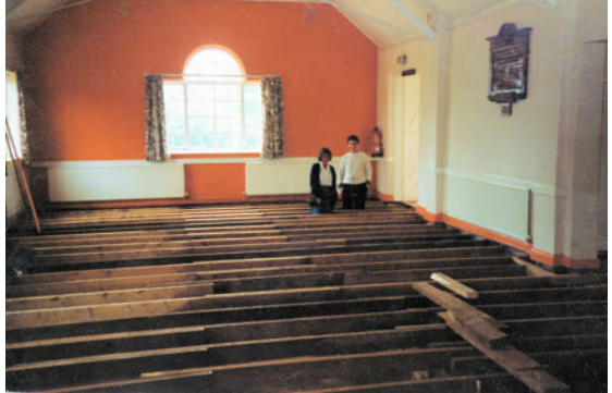
1988 old floor removed
