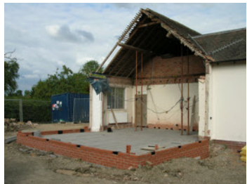
Extension in progress
