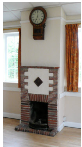
One of the two original fires heating system
