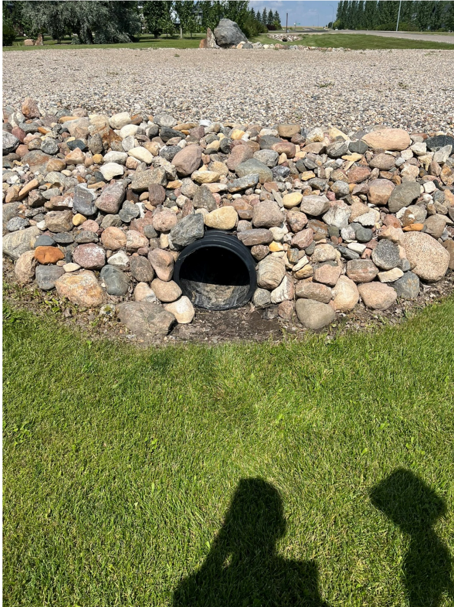
Figure 3: An example of a clean culvert
