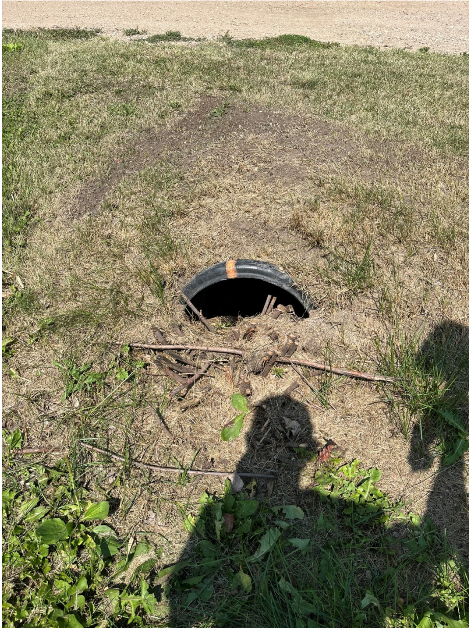
Figure 2: Another example of a filled in culvert end
