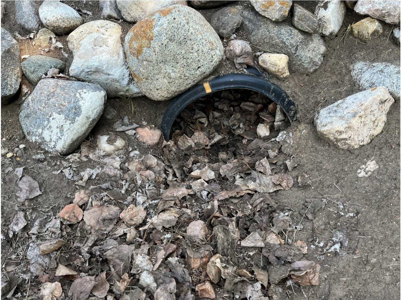
Figure 1: An example of a filled in culvert end
