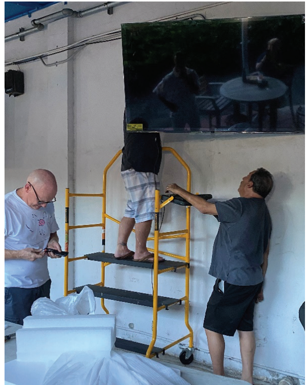
Installing new patio TV
