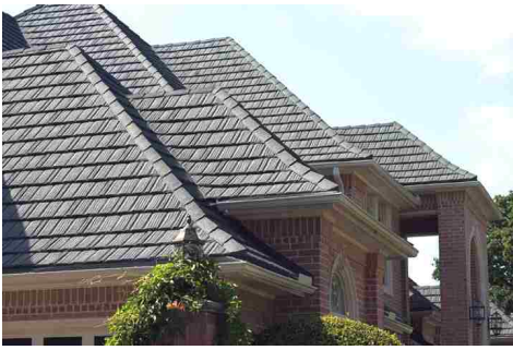
A Stone-coated Steel Roof – one of the ACC's newly approved options for TOS residents.
