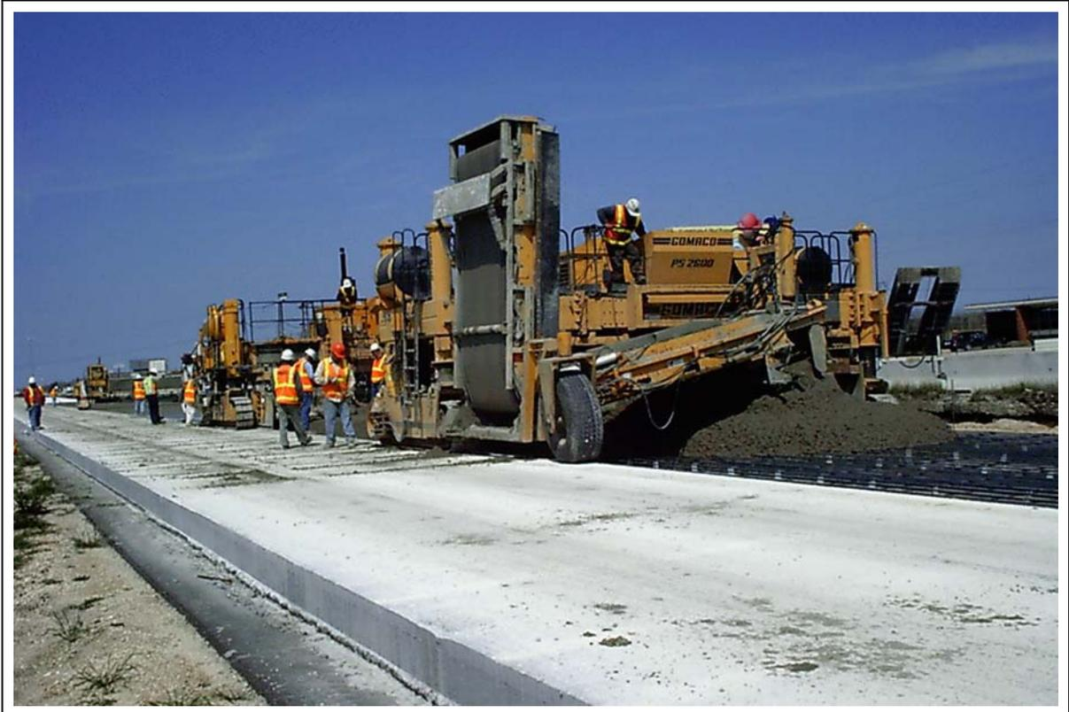
FIGURE 3: Steel Ahead of Placer on IH 10, Texas, U.S.A.
